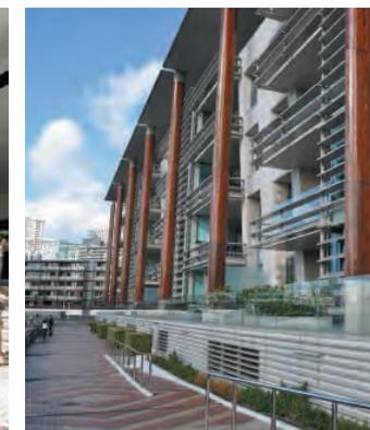
Facia treatment where ground floor is raised above finished footpath level
